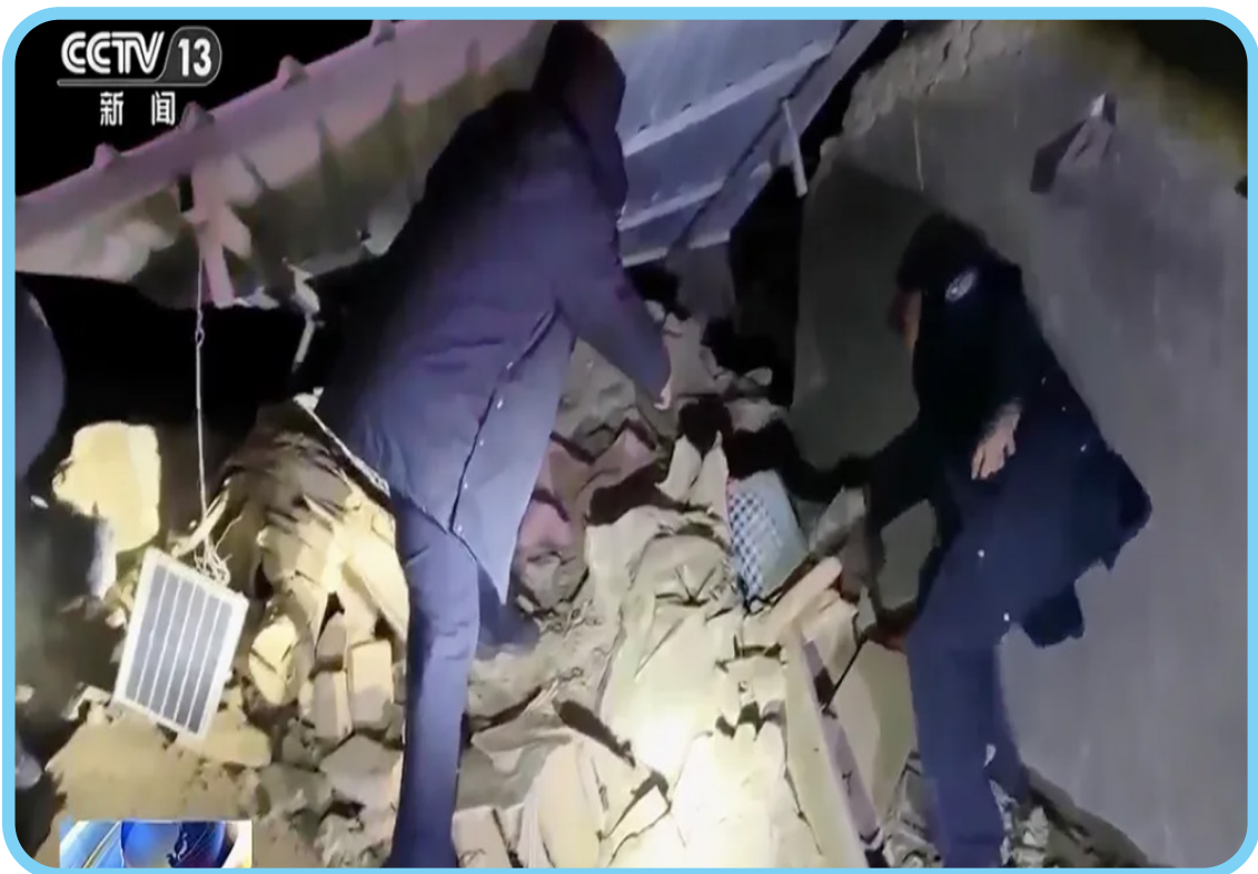
A screengrab of footage from CCTV shows rescuers working in rubble.
