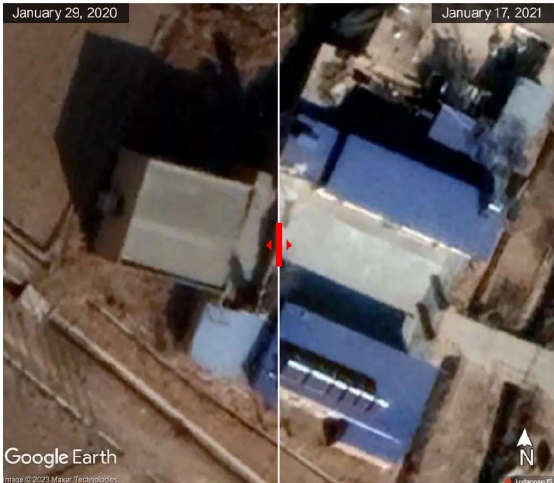
January 29, 2020: © Maxar January 17, 2021: © Maxar Liaoqiao South Mosque's main hall was demolished between January and August 2020.
